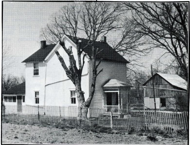
The Ed Schroeder Home north of New Melle
